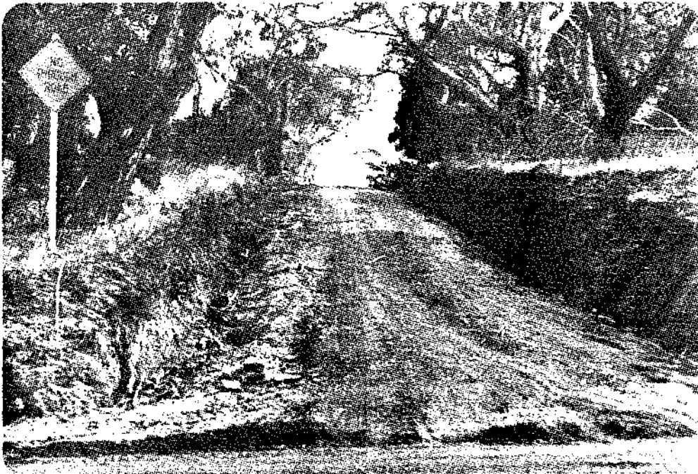
Photo 10 : Corner of Pearse Road and Aireys Street. A poorly constructed and surfaced road subject to severe erosion.
