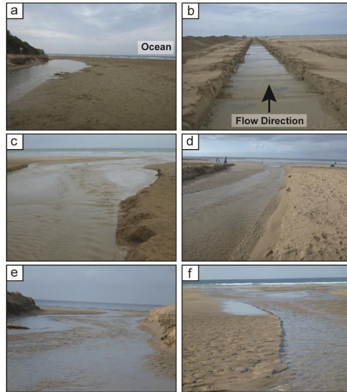
Figure 6. Photos of Anglesea artificial opening. (a) Closed estuary immediately prior to entrance opening 14/02/2014; (b) Channel excavation 10 am 14/02/2014; (c) Initial growth of lower entrance channel spit 16/02/2014; (d) Further spit development 17/02/2014; (e) Spit growth and a reduction on outflow depth 18/02/2014; (f) Further bar elongation and berm accretion 19/02/2014 prior to full entrance closure. All images taken at low tide.
