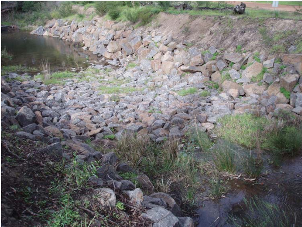
Figure 3.3 Rock chute installed downstream of Old Coach Road bridge
