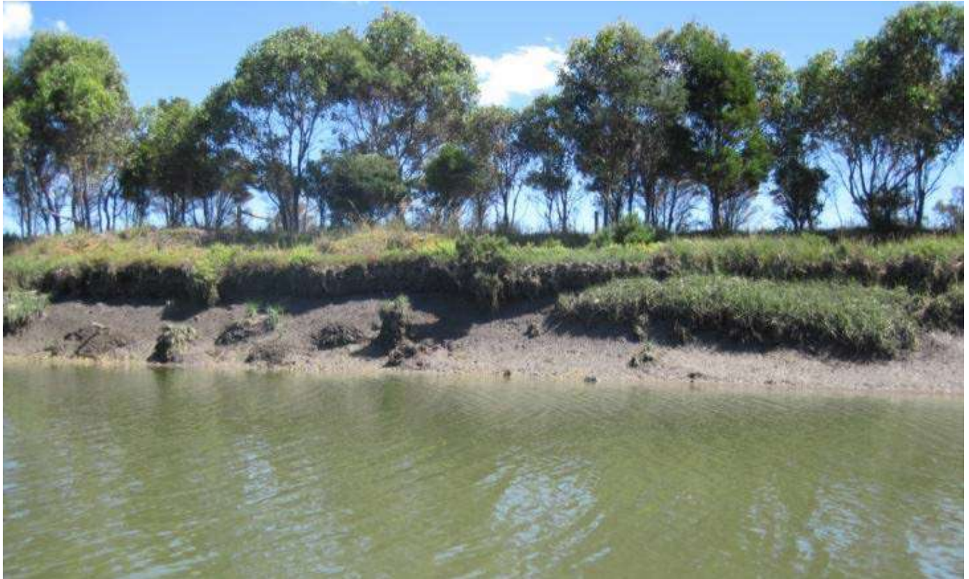
Figure 50. Bank erosion and slumping along the Bass River estuary.
