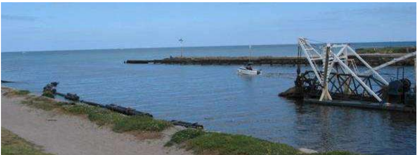
Figure 27. Training walls and dredge at Mordialloc Creek estuary.
