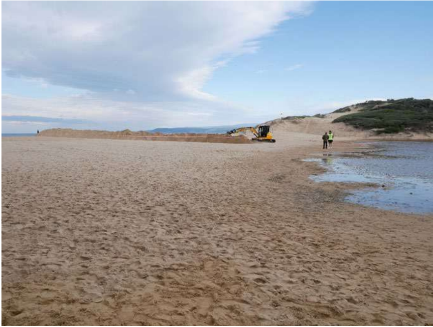
Figure 2.8: An artificial estuary opening where a channel is dug from the ocean, through the berm to the estuary basin at Painkalac Creek, Aireys Inlet, Victoria, June 2020.
