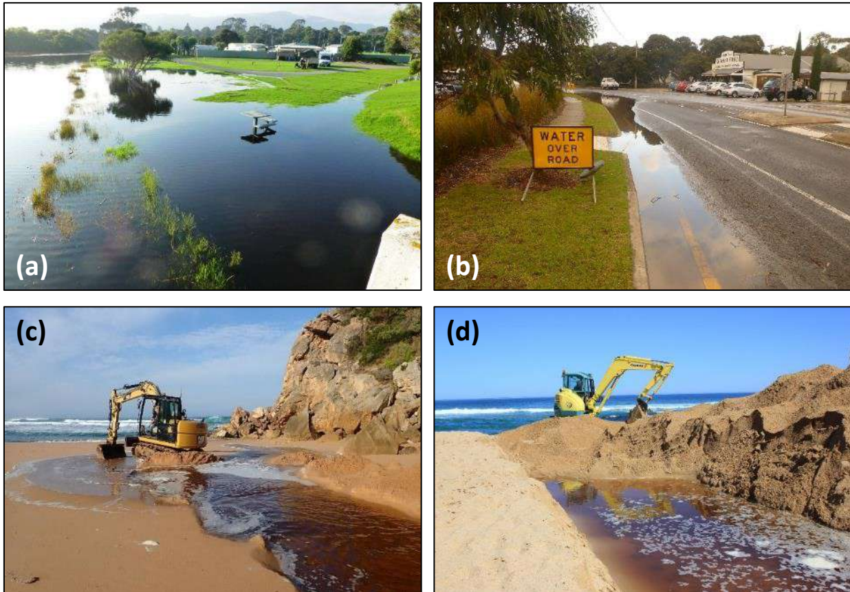
Figure 1a-d. (a) Flooding at the Barham and (b) Anglesea River estuaries prior to artificial opening; (c-d) artificial openings being undertaken at the Gellibrand River estuary. Photos from EstuaryWatch (2019).
