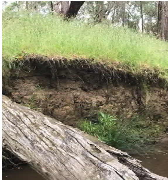
Figure 2.7. Looking across Painkalac Creek at freshly exposed soft sediment face, just below the dam outlet.
