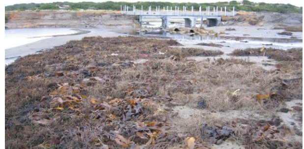
View of the new culverts during construction
