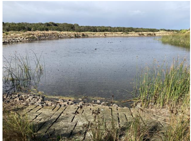
Stormwater pond adjacent to wetland
