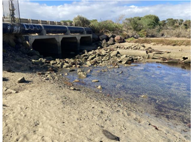
View of the culverts connecting Mullet Creek to the estuary
